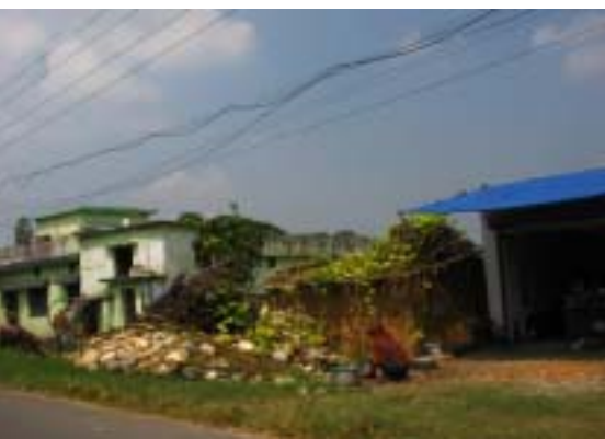
Supporting sustainable development
