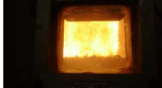
Waste combustion inside the incinerator
