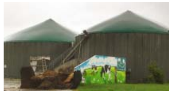
Two wet fermentation digesters.
