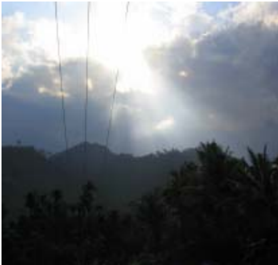
Transmission wires near Agali
