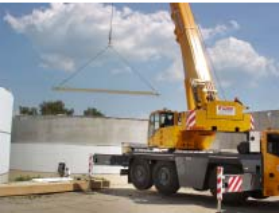
Final positioning of a wooden truss of the digester's roof.
