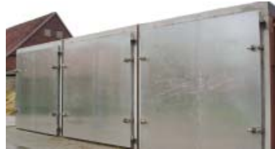
Dry fermentation digesters
