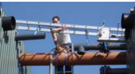
Biogas pipe fixing for the digester
