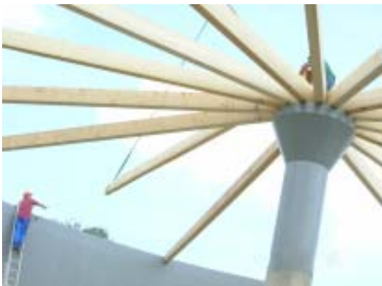
Mounting of the "biogas dome".
