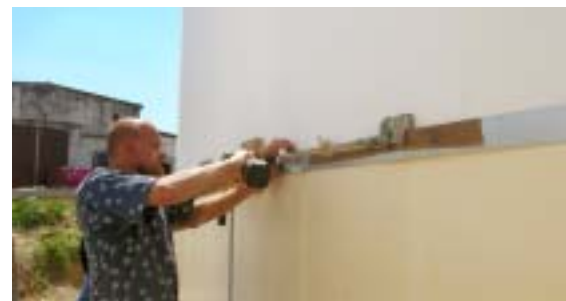
Providing insulation for digester
