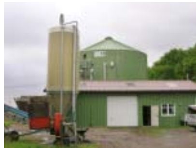
Wet fermentation digester
