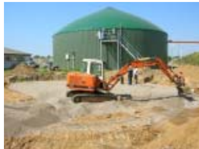
Ground preparation for digester construction work
