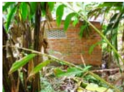
Powerhouse in Nedumkandam
