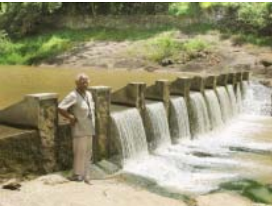
Mr. Thomas in front of the potential intake-weir.
