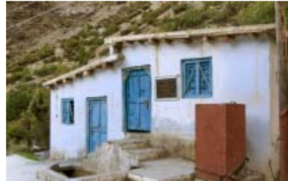
Powerhouse in Malari
