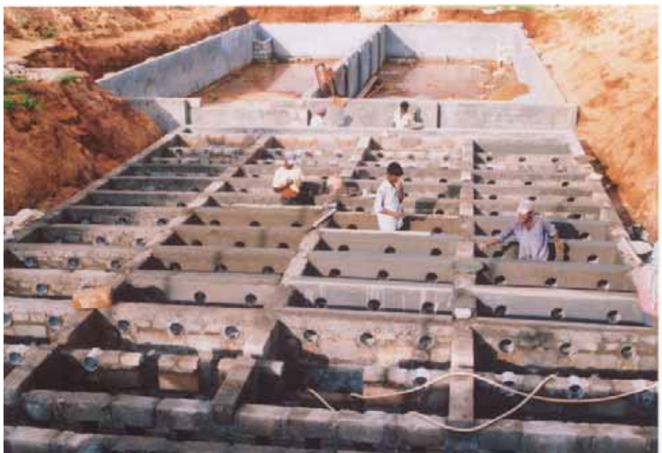
Construction of an anaerobic baffled reactor
