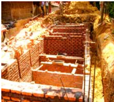
The DEWATS modules for physical and biological wastewater treatment in schools are: bio digester, sedimentation chamber, anaerobic baffled reactor and discharge to drainage ditch.
