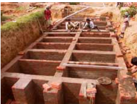
DEWATS plant for an apartment block (above) and under full construction (below)
