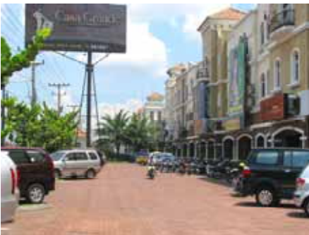
The surface of the decentralized underground DEWATS system can be used as parking space.
