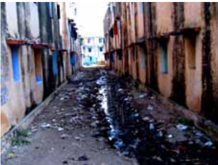
Discharge of untreated wastewater into the street: a consequence of missing connections to a central sewerage system.
