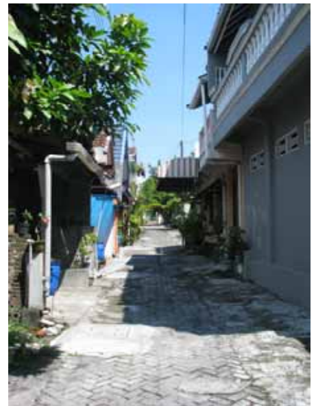
The units of the DEWATS plant are installed underground. Therefore, the system is nearly invisible.
